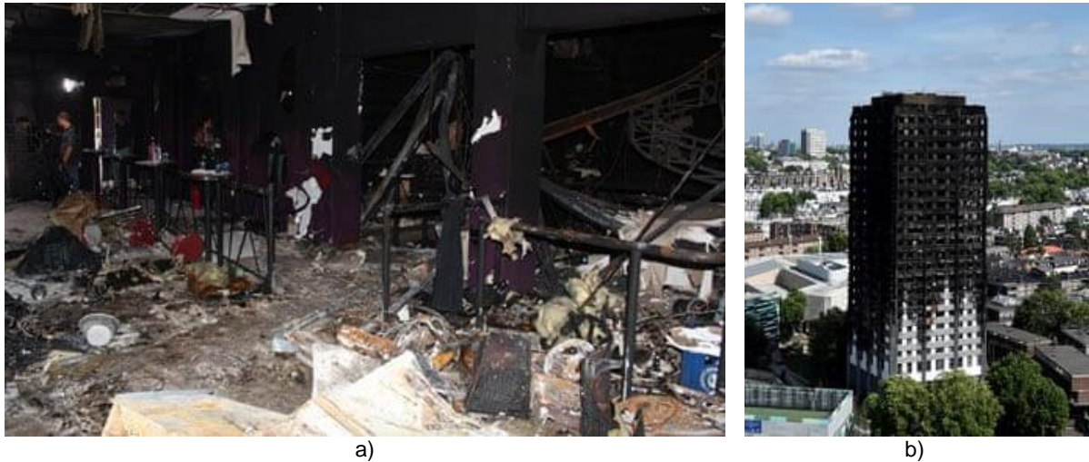
Figure 1: Kiss Nightclub (a) and Grenfell Tower (b) after the fire incidents (source: Reuters)
