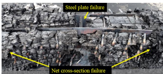
Figure 11: Failure mode of connection n°11'
