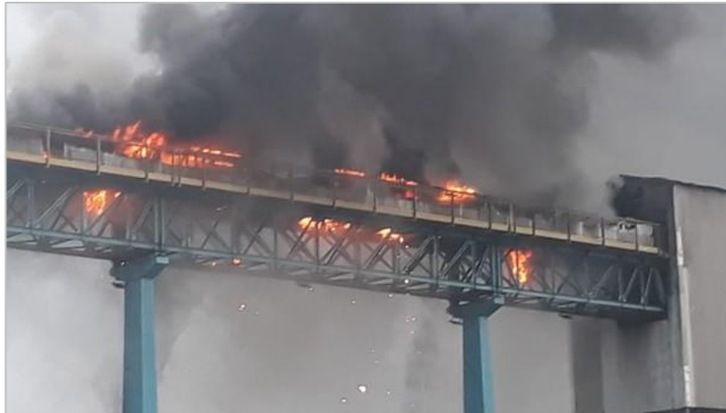
Figure 1: Fire in a conveyor in Santos Harbor (Portal G1, 2019) [6]
