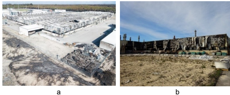
Fig.1 – Damages in the building envelope in industrial sites affected by 2017' Greatest Forest Fires in Portugal [3]
